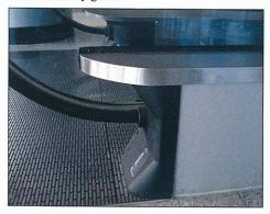
Extended deck cover over the handrail safety guard is designed to prevent accidents at the inlet of handrail.
